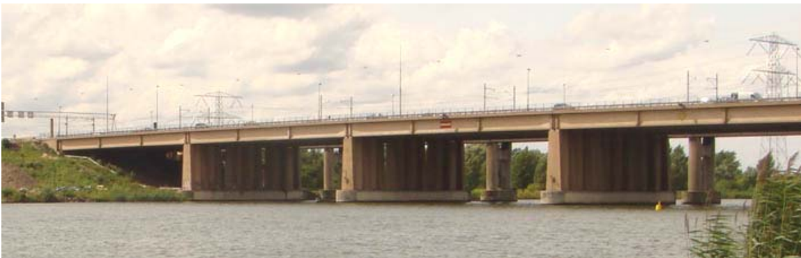
Fig. 1: The Hollandse Bridge: Currently subject to a monitoring project.
