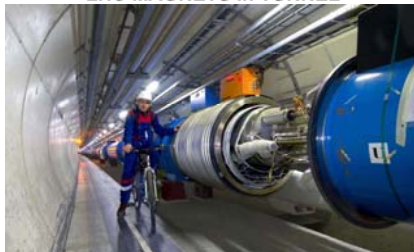
MAGNETS and CRYO-SUPPLY-LINE (He 4.2 K) REAL 8 th 16 th Erik HEIJNE CERN PH Department Veldhoven 17 November 2005
